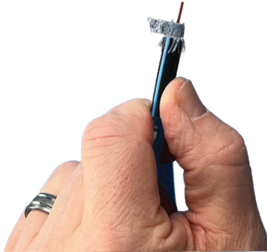
Figure 59: Cutting the inner foil
