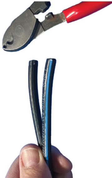
Figure 51: Splitting the IFL cable to length
