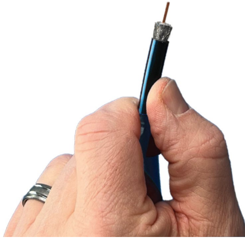
Figure 57: Exposing the braid and foil
