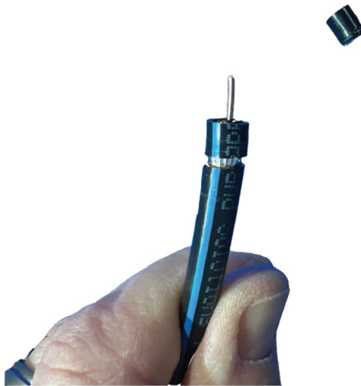
Figure 56: Exposing the center conductor
